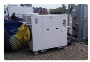
Nminal cooling duty: 50 kW Nominal heating duty: 100 kW Air flow (max): 11,500 m<sup>3</sup>/h
