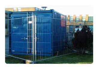
Nominal heating duty: 300 kW Power supply: 240 V 1 ph N+E 50 Hz Noise level: 55 dBA
